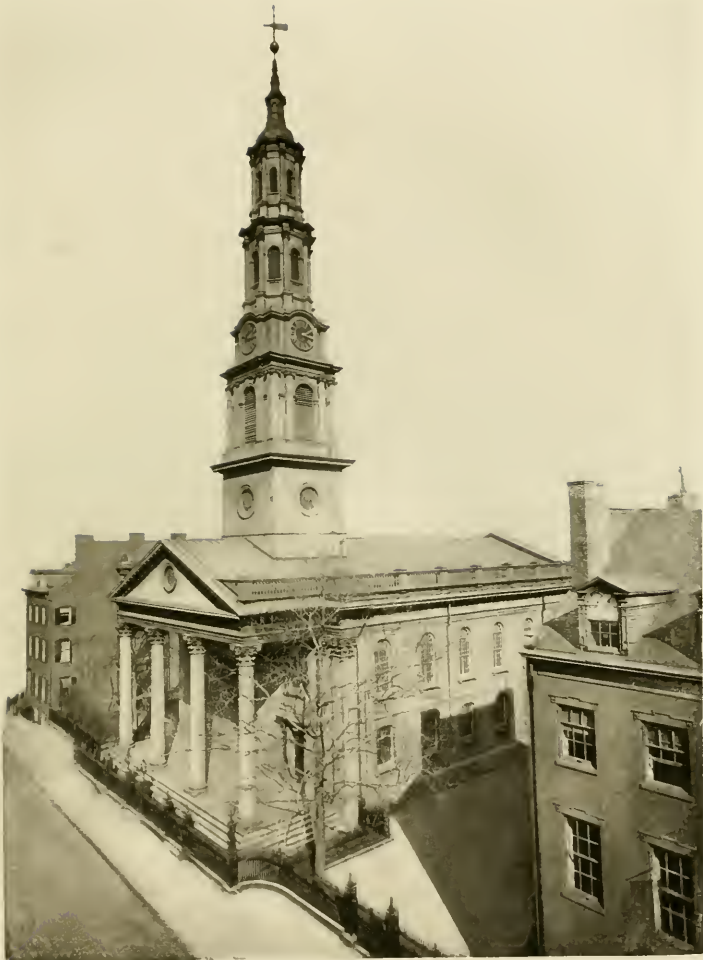
St. John's Chapel was commenced in 1803, completed in 1807 and consecrated that same year. It has been three times altered or enlarged.
